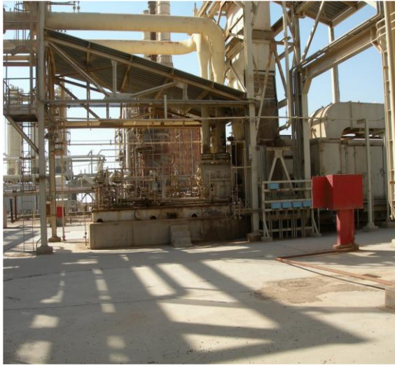
K03 Compressor Repair
